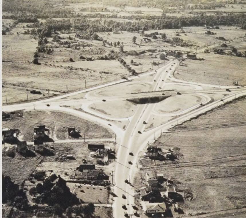
1928 Construction of the first “clover leaf” at Routes 1&9 and Route 35 in Woodbridge.
